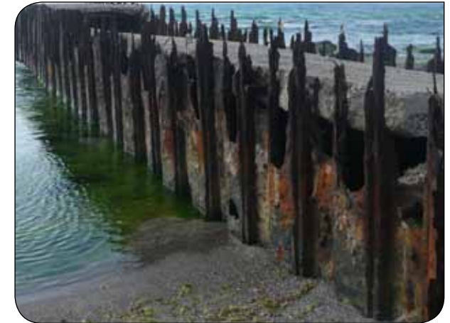
Sheet Piles made of Steel
